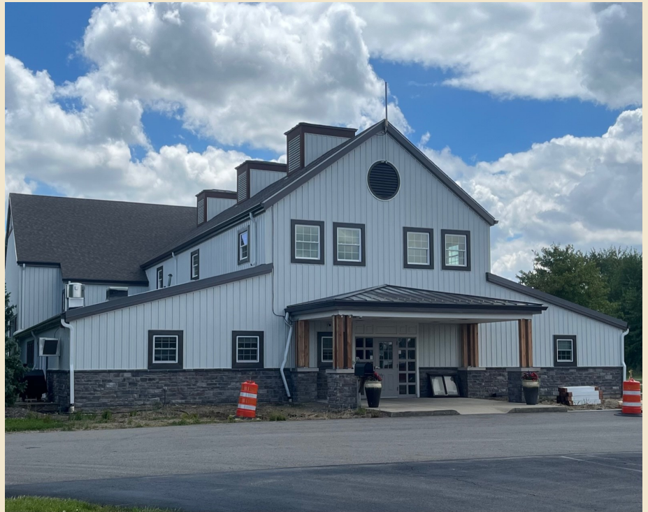
Above: New windows, siding, and trim combine to create an updated color scheme. The new steel siding and aluminum trim are expected to provide better protection and longevity than the original vinyl products that had reached their end of life.
