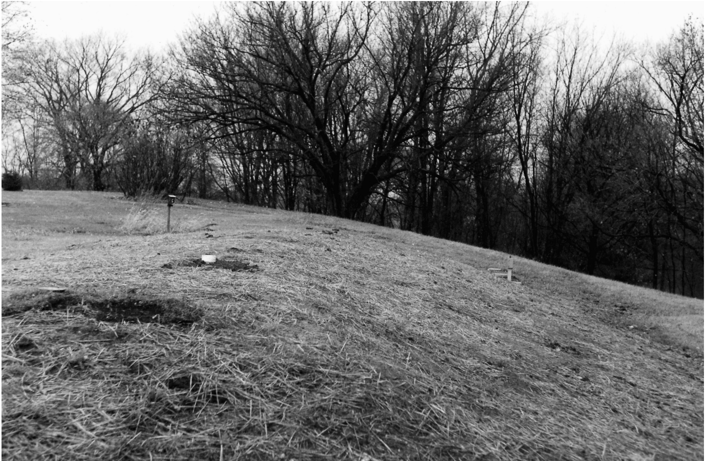
Newly constructed mound system to serve three-bedroom house.
